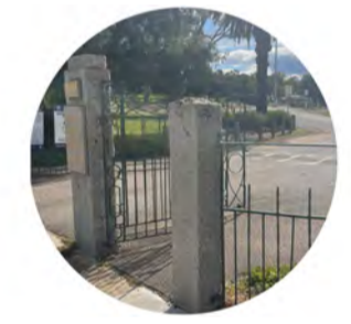
MATERIAL PALETTE TO BE COMPLIMENTARY TO THE ENTRANCE PILLARS TO THE SITE, SUCH AS THE USAGE OF STONE AND GREY TONED MATERIALS
