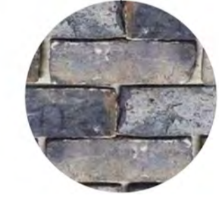
OPPORTUNITY TO USE RECYCLED BRICKS FOR THE NETBALL COURT RETAINING WALL
