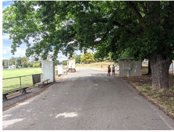
Figure 4.22 View looking south, towards hill. Public amenities block (right) and coaches' boxes (left) proposed to be demolished.
