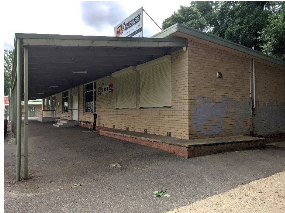
Figure 4.18 Existing Castlemaine Football and Netball Club Pavilion.
