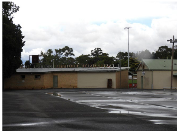
Figure 4.39 Rear elevation of existing pavilion.
