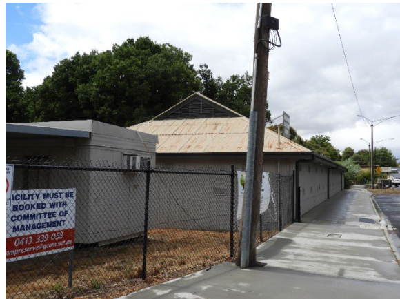
Figure 4.24 Agricultural building and south end of freestanding office; Forest Street boundary.
