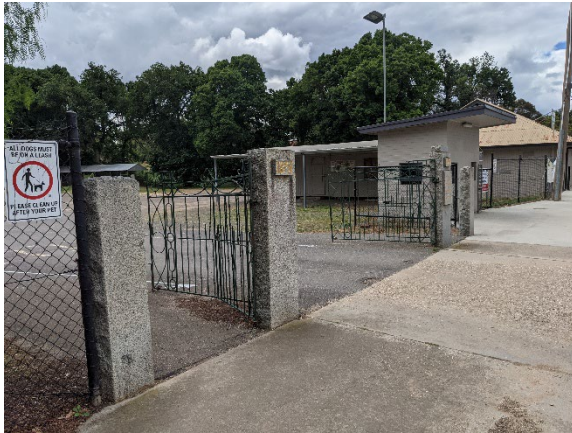
Figure 4.25 Centenary entry gates and ticket box, both to be retained (front).
