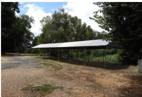
Figure 4.29 Sheep pen, one of two, on the east side of the reserve. To be retained.
