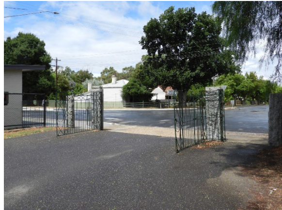
Figure 4.26 Centenary entry gates and ticket box, both to be retained (inside view).
